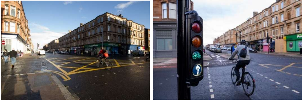
Before (Left: 2016) and after (Right: 2023) the construction of the South City Way. Credit: Sustrans (Left) & John Linton (Right)
