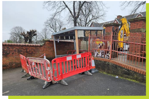
Figure 1: Construction of bike shelter with eco roof. ©Vale of Glamorgan Council
