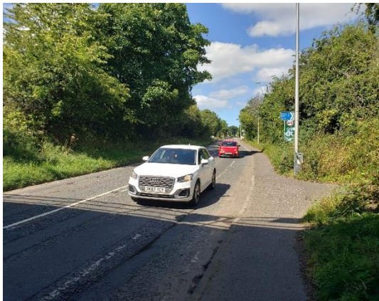
Existing ramp joining Old Dalkeith Rd
